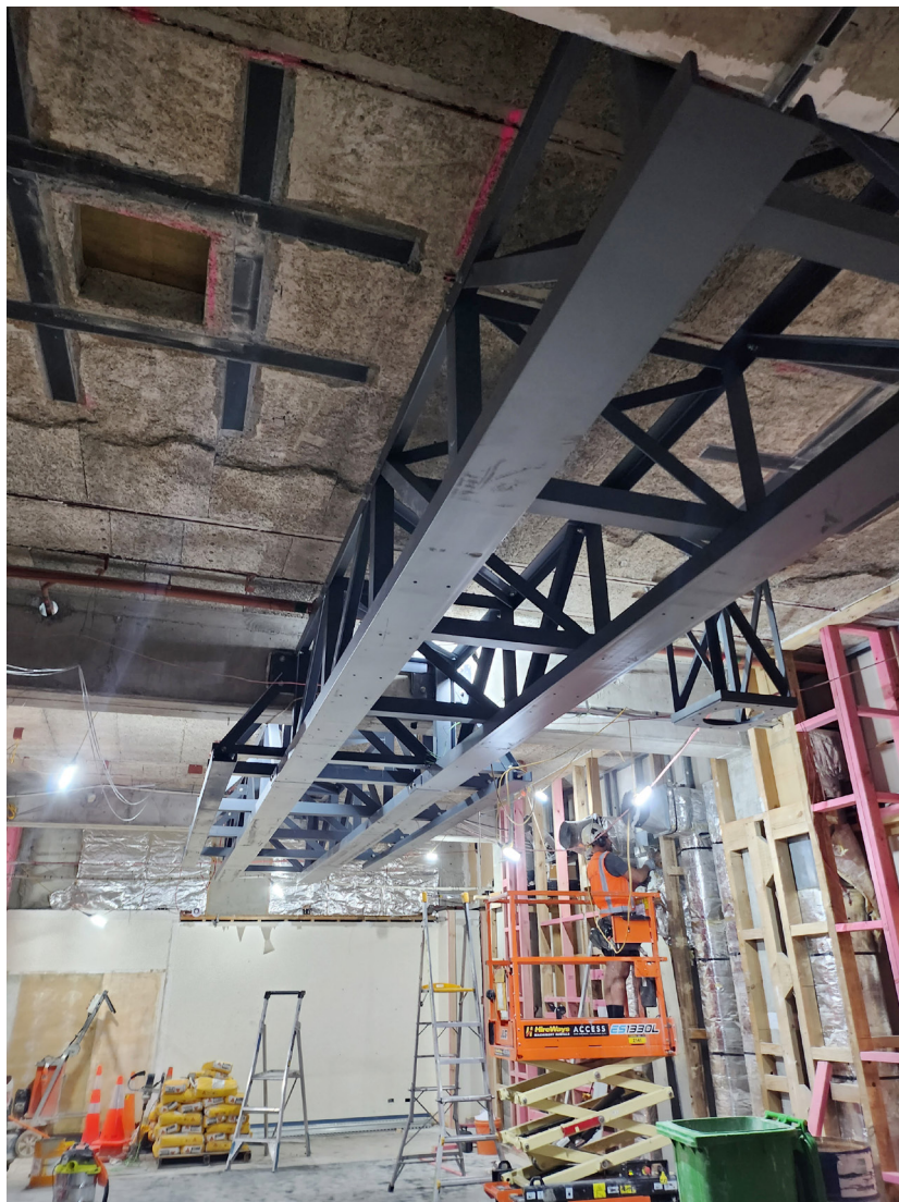
Gantry in place on which the cath lab will be hung.
