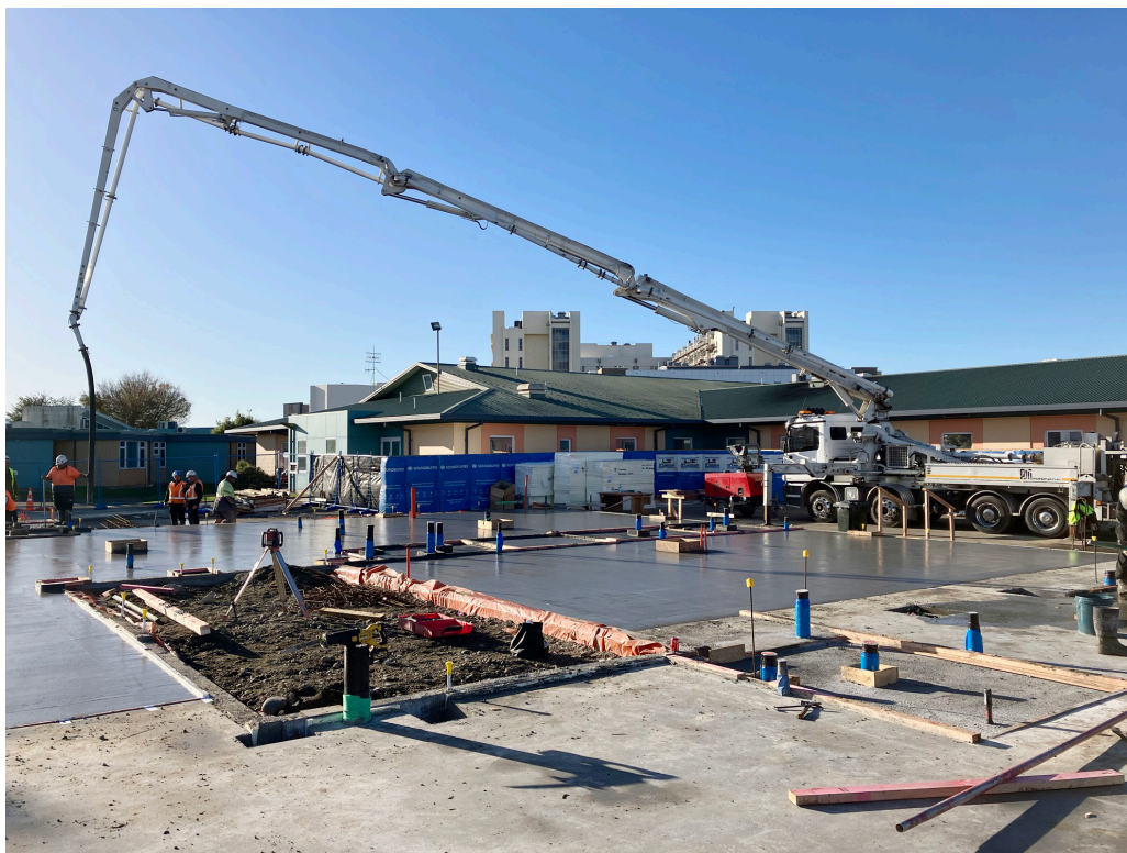
AMHU concrete floor Stage 1 poured.
