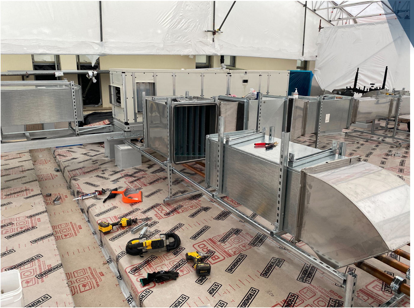
Installing plant on the rooftop.
