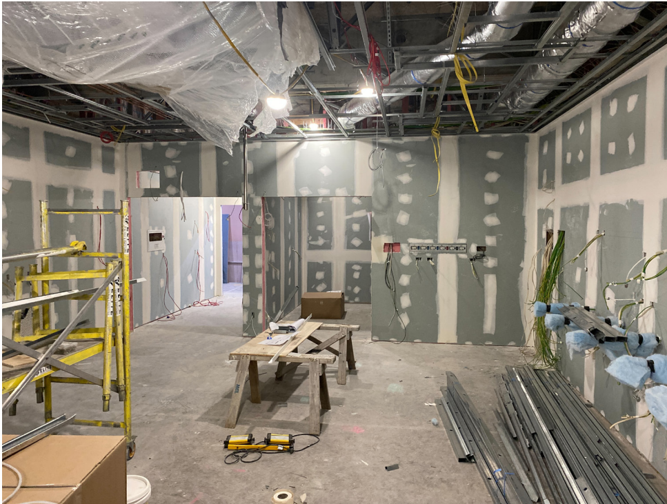
SPIRE electrical and other key services progressing.
