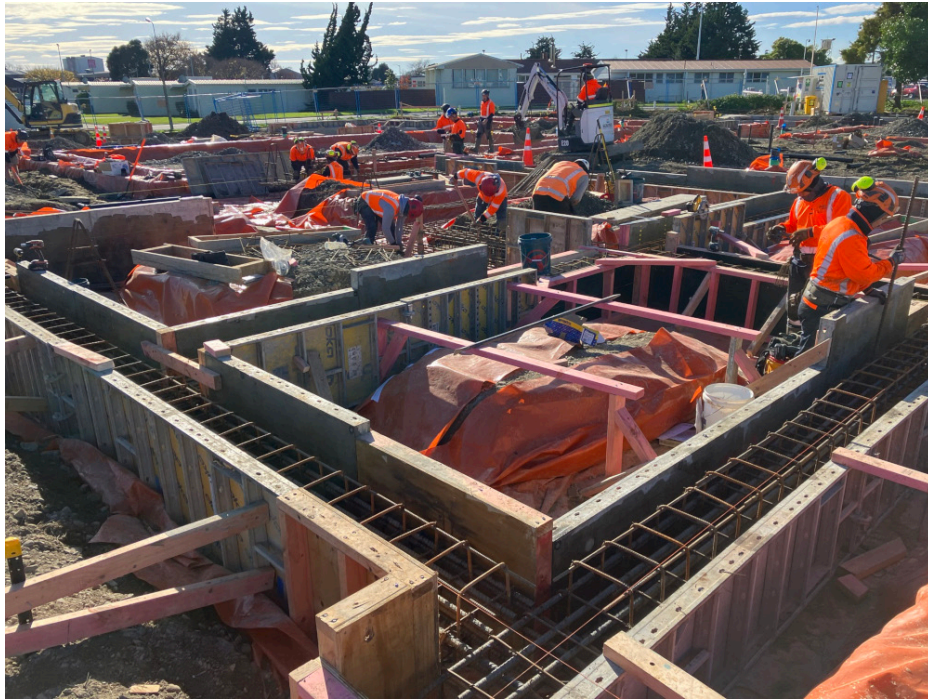
AMHU foundation works in progress.
