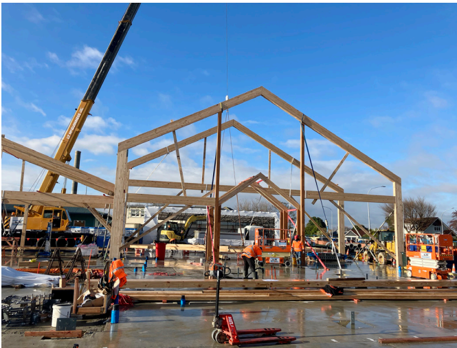
First section of framing slowly rising from the ground up with support from the on-site construction crane.
