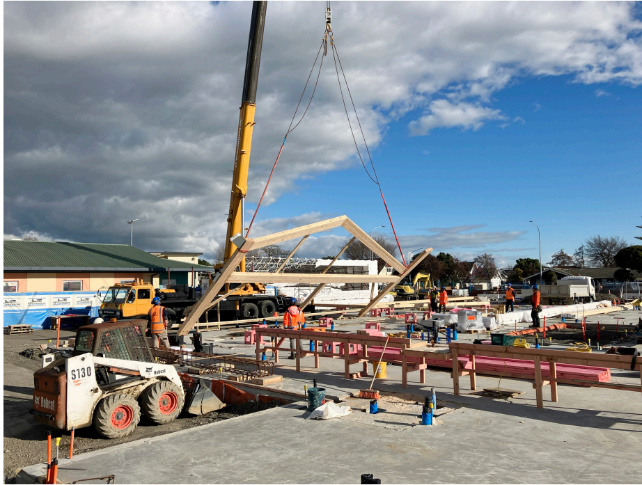
First section of framing slowly rising from the ground up with support from the on-site construction crane.
